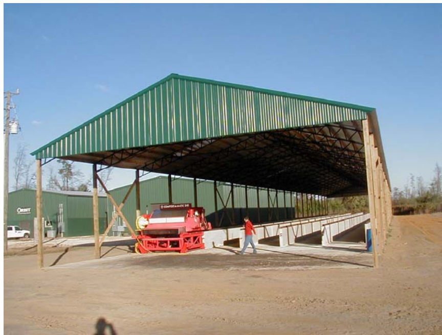
Figure 2: Super Soil solids processing facility installed at Hickory Grove farm in Sampson County, NC.
