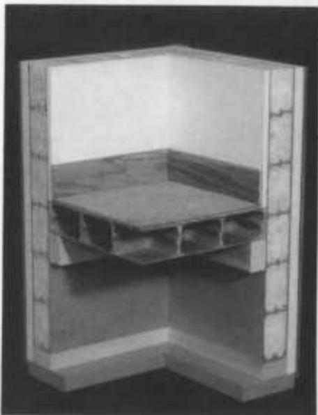
Uses for wood fiber panel products include insulating acoustical board; carpet board; wall, ceiling, and floor acoustical insulation panels; nail base board; and floor and roof insulation boards.
