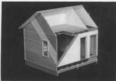
The Spaceboard construction technique yields products that can be made thin enough for strong, lightweight walls and floors.
